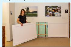
**Removable wainscotting** panels can be washed and disinfected after a flood. They are easy to remove and the insulation is FEMA rated foam and can also be pulled out, washed, and replaced.
